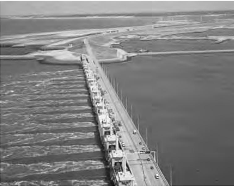
*Figure 13. The 3 km long storm surge barrier Oosterscheldekering
