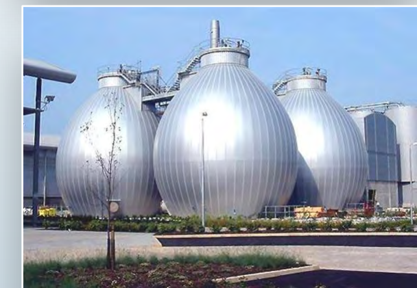
SLUDGE DIGESTORS
