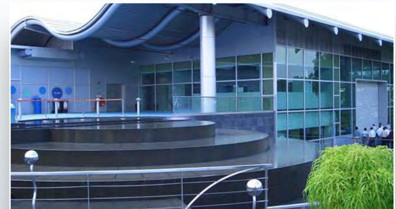
NEWATER INSTALLATION OF PUB IN SINGAPORE
